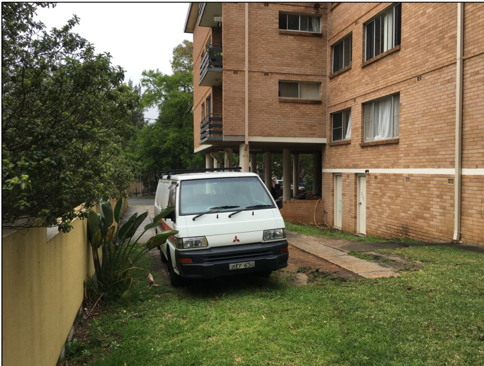
Figure 2: View looking to the south from eastern side of building
